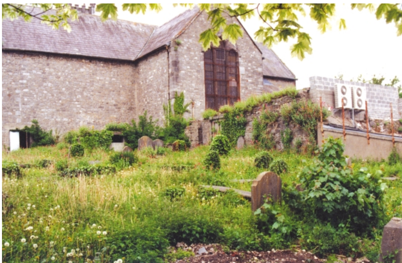
Plate 15: Inappropriate use of the boundary wall to the rear of the Kieran Street properties
