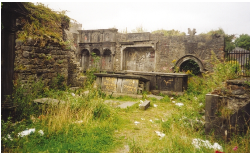
Plate 12: Vandalised area at the east of the Church (behind the hoarding)
