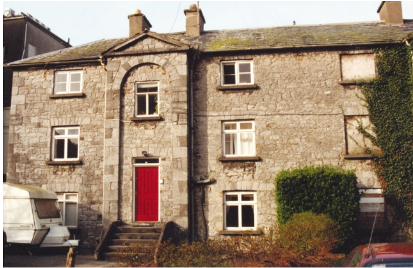
Plate 20: The occupied Almshouse
