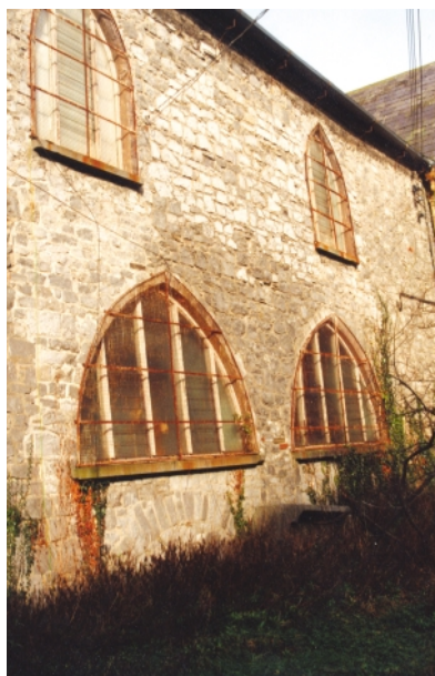
Plate 31: Security mesh on windows
