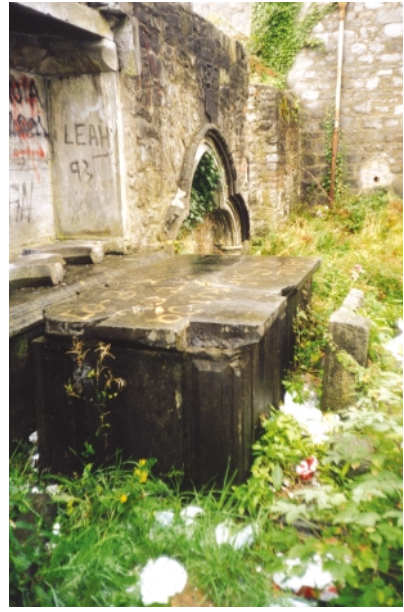
Plate 17: Destroyed altar-type monument to the east of the Church
