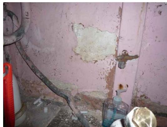
Fig.35: Effloresce and rising damp at low level to the west wall.
