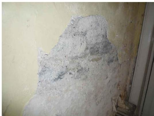
Fig.74: Failed plaster to the west wall.
