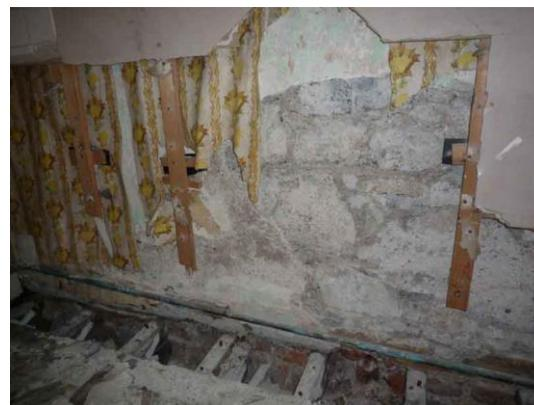
Fig.104: Failed plaster to west wall beneath dry lining.
