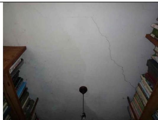
Fig.31: Cracking of ceiling plaster.
