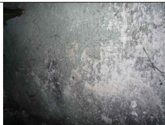
Fig.94: Penetrating damp to the east wall.
