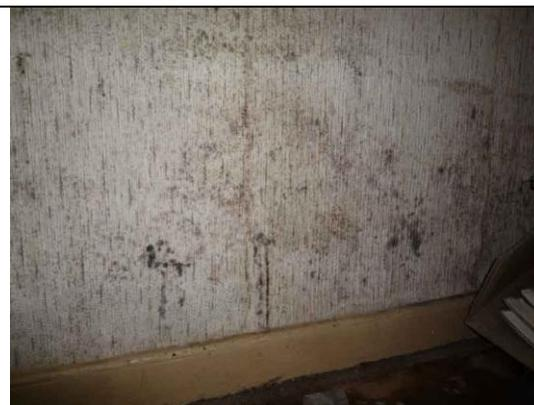
Fig.4: Rising damp at low level indicating excessive levels of moisture within the structure.
