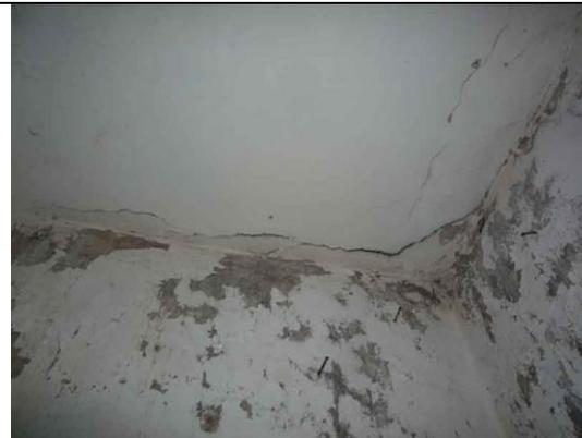
Fig.20: Cracking to ceiling at junction with south wall.
