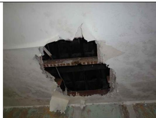
Fig.102: Hole to ceiling plaster.
