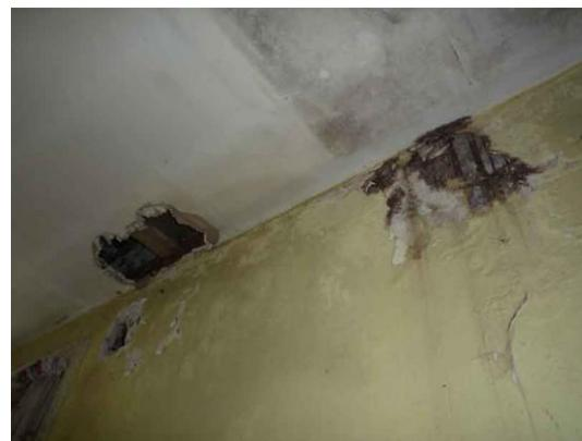
Fig.90: Hole in ceiling and penetrating damp at high level to north wall.
