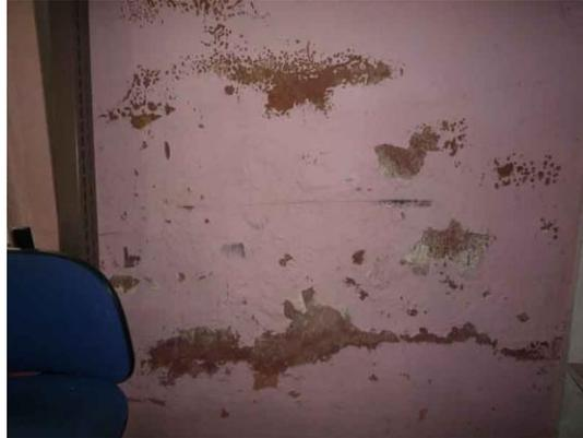
Fig.25: Plaster failure to the east wall indicating rising damp.
