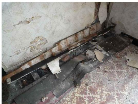
Fig.99: Missing timber floorboards to the east wall.
