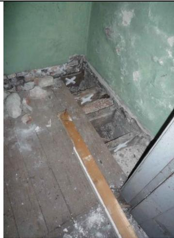
Fig.66: Missing floorboards, timber skirting and failed plaster to room F07.
