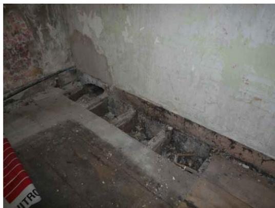
Fig.57: Missing timber floorboards to east.
