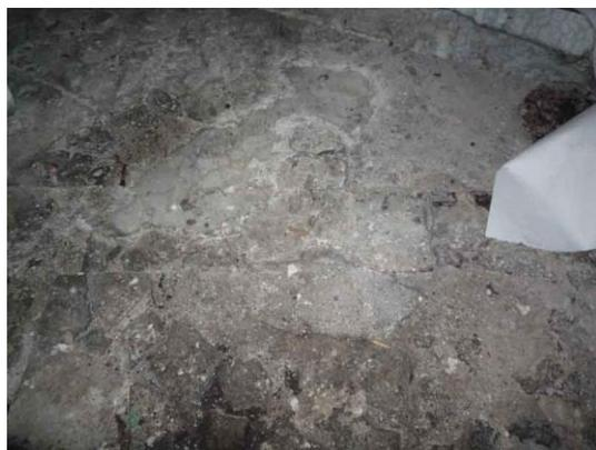
Fig.13: Broken-up concrete floor.
