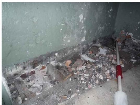
Fig.91: Missing floorboards to the north wall.
