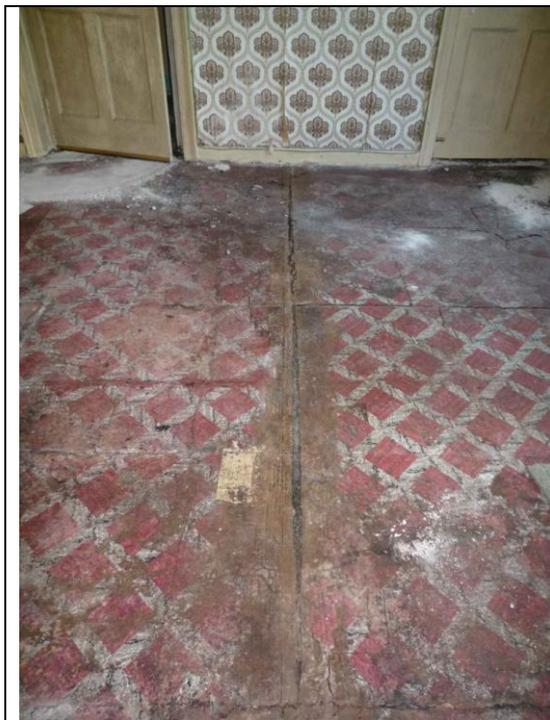
Fig.45: Linoleum floor covering to the limestone flags.
