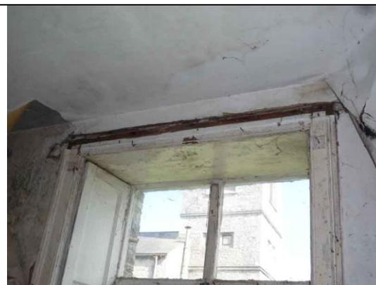
Fig.48: Missing section of architrave to window opening.
