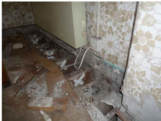
Fig.80: Missing floorboards to south wall.
