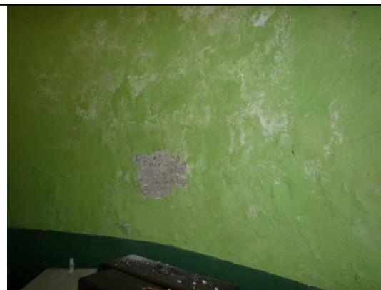
Fig.37: Efflorescence and plaster failure to east wall.
