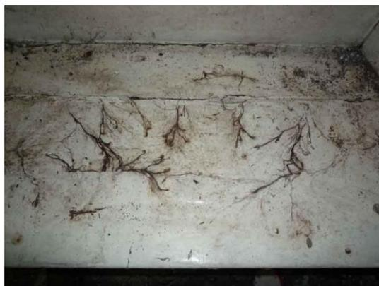
Fig.40: Fungal growth to window cill to easternmost opening.
