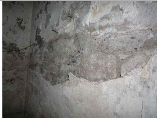
Fig.19: Failed plaster to the west wall.
