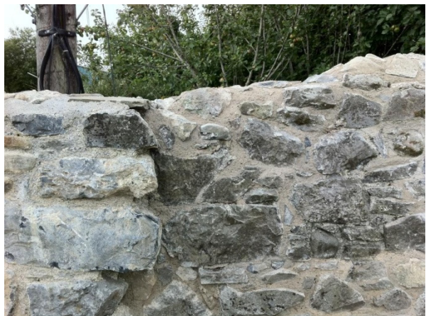
Detail of the repointing work. Samples of sand and exemplars of pointing were agreed in advance.
