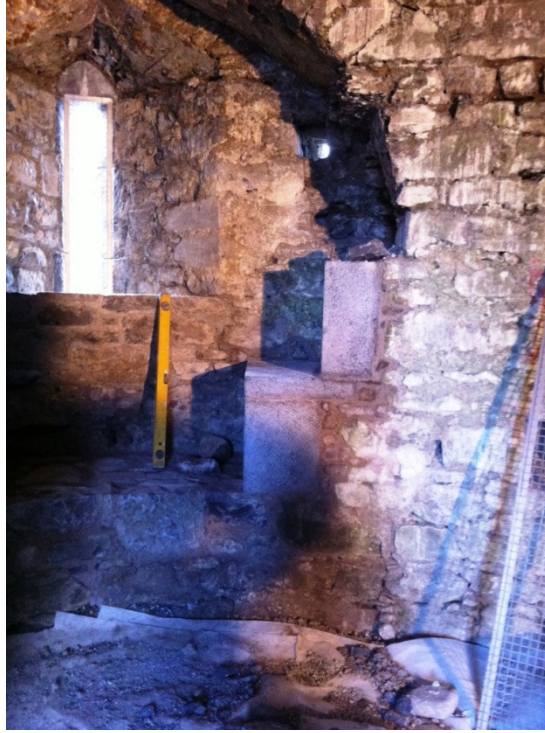
Loop No. 135 during rebuilding of stone seats
