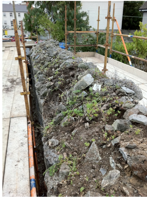
There was extensive vegetation and soil on the wall top. This was carefully removed.
