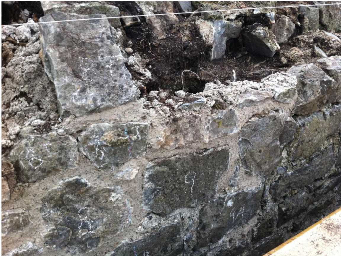
Victorian facing stones are numbered removed and reinstated
