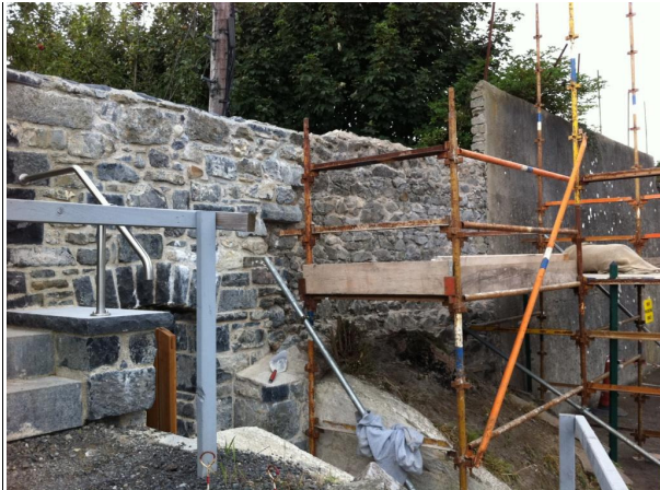
Repointing work underway
