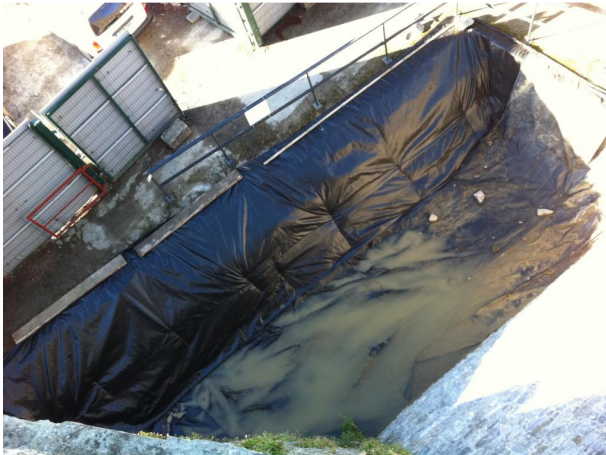
The ditch will be completely protected over the winter with heavy duty membrane, fixed at the top and pinned into the face of the ditch.
