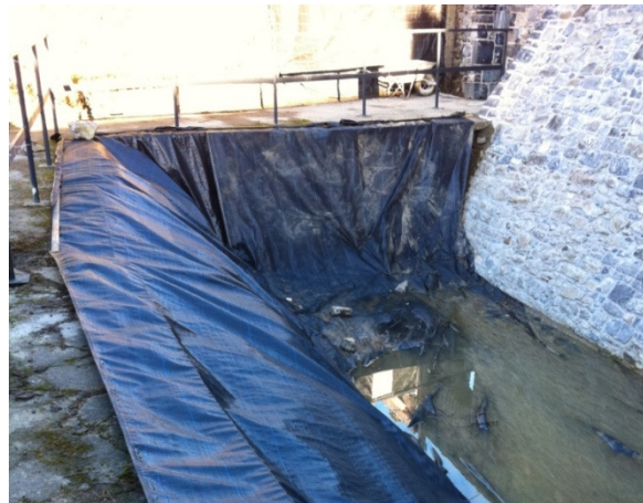
The ditch will be completely protected over the winter with heavy duty membrane, fixed at the top and pinned into the face of the ditch.
