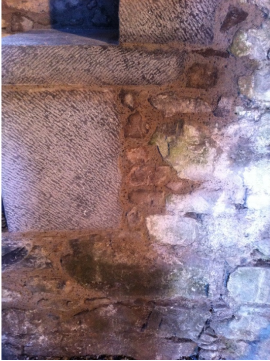
Loop No. 135. Detail of stone tooling and adjacent rubble stonework
