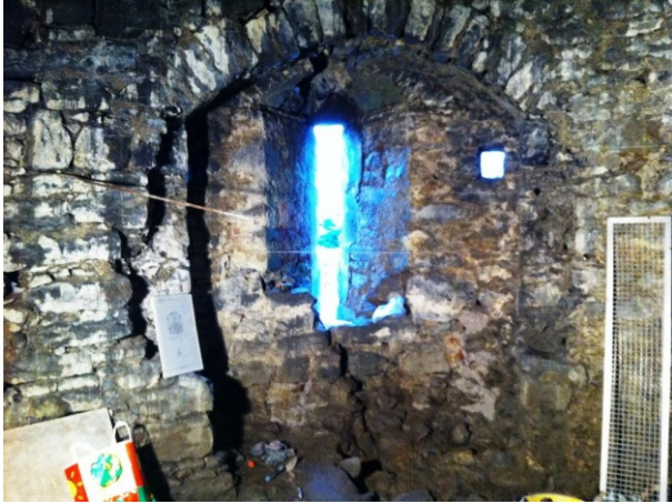
Loop No. 145. Surveying underway, before rebuilding commences
