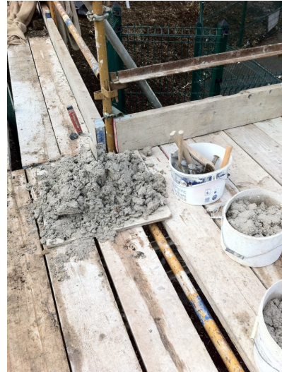
Fresh mortar ready for application
