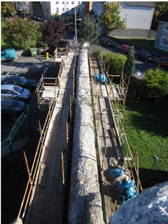
The completed wall top left, and right, protected from inclement weather
