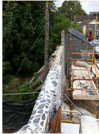
View of the repaired wall top.
