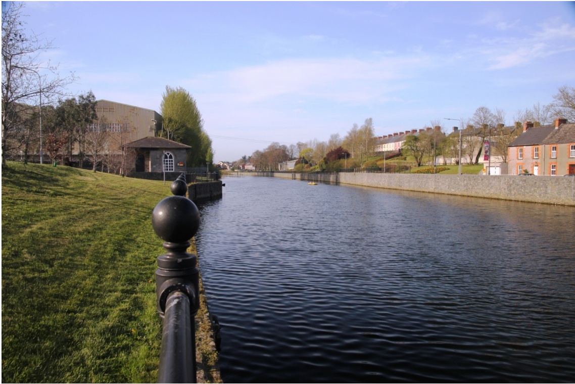
Plate 3 Upstream of proposed pedestrian bridge location.
