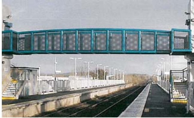
5 - Vierendeel Half Through Truss (Portlaoise)
