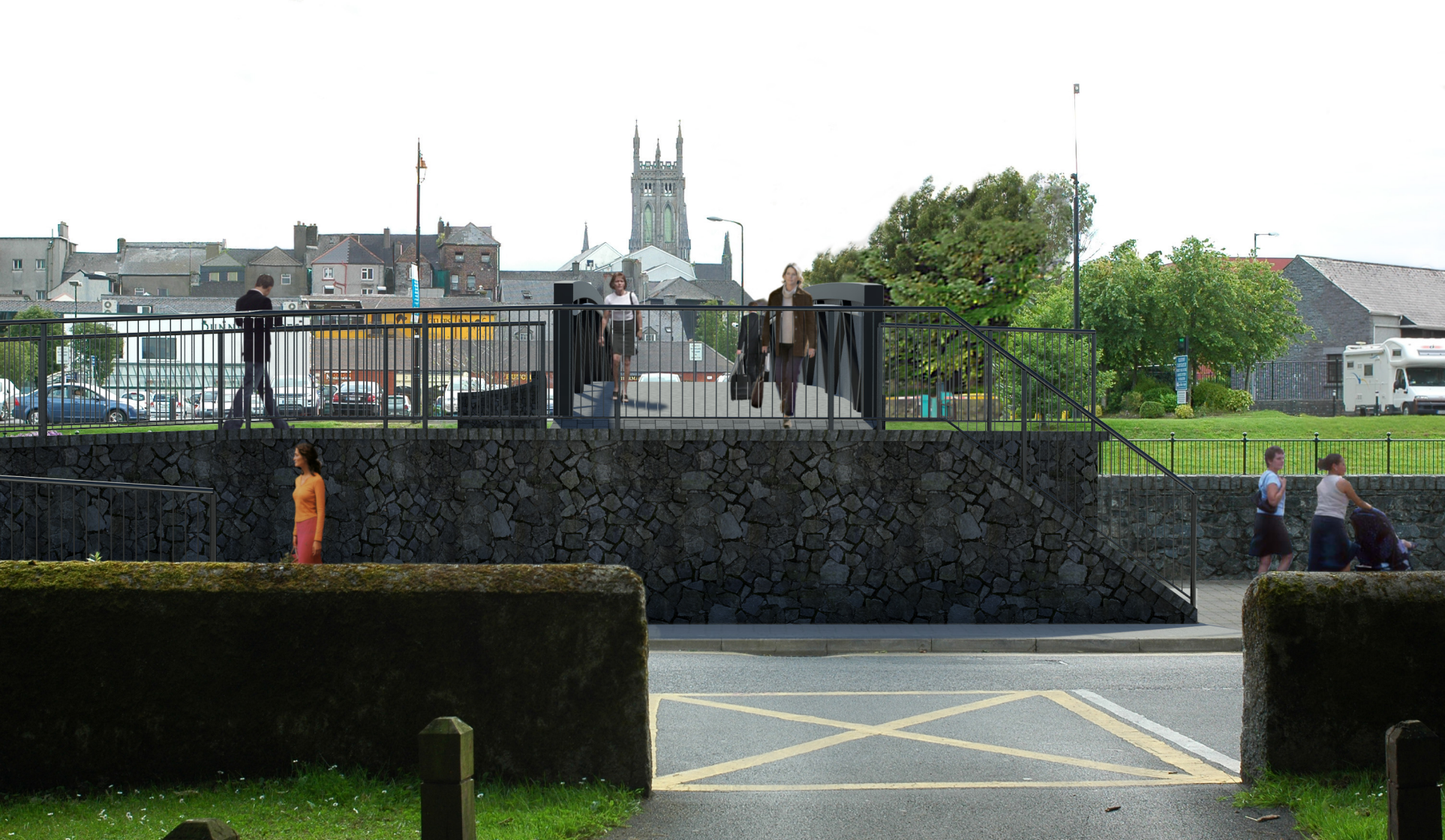
Kilkenny City Pedestrian Bridge. View 3 – East Bank (Johns Quay)
