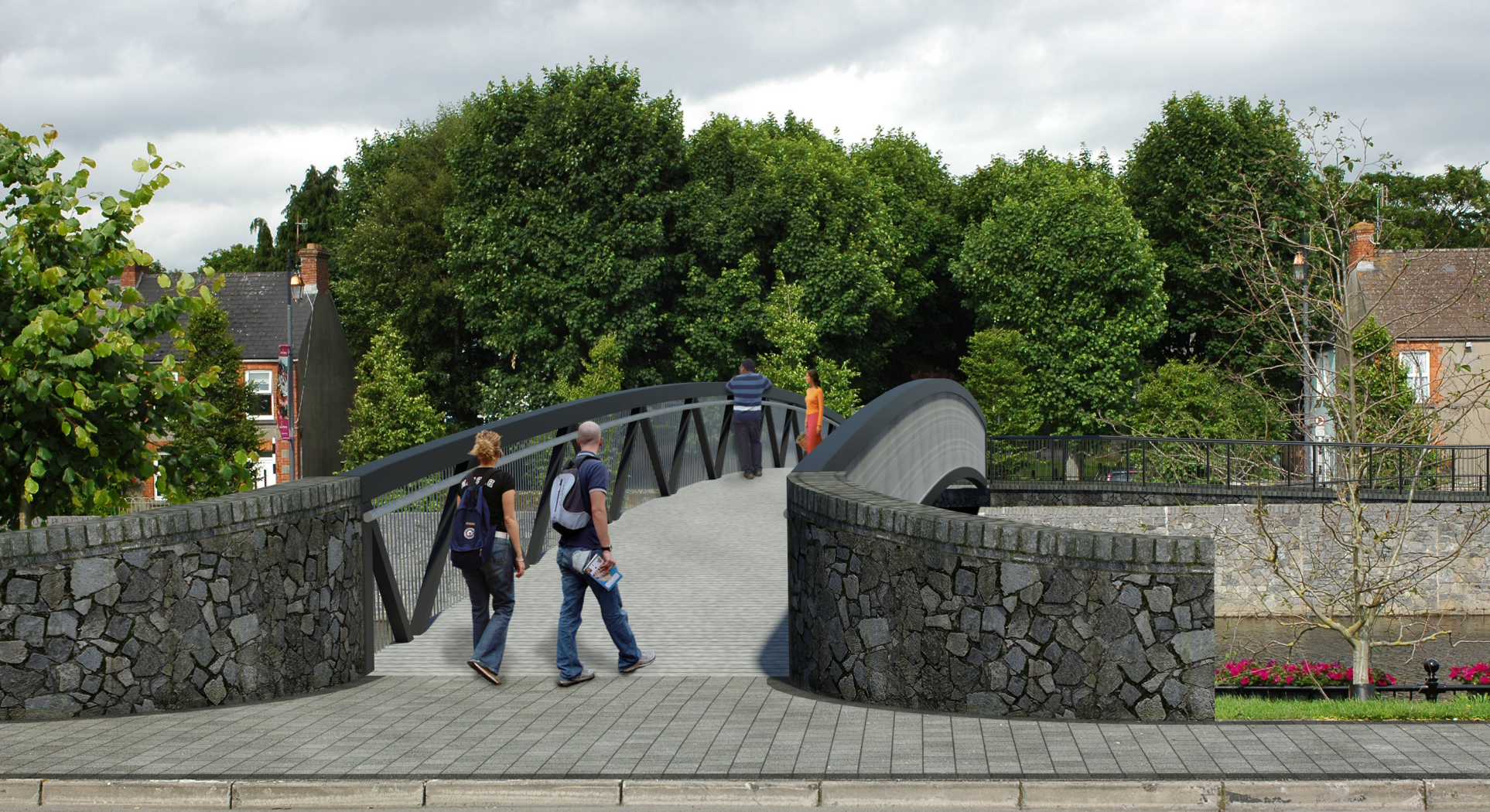
Kilkenny City Pedestrian Bridge. View 2 – West Bank (Bateman Quay)
