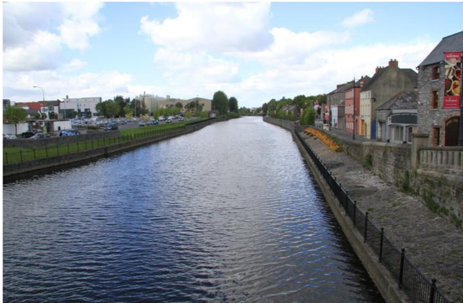
Plate 11: View upriver from John's Bridge towards Green's Bridge
