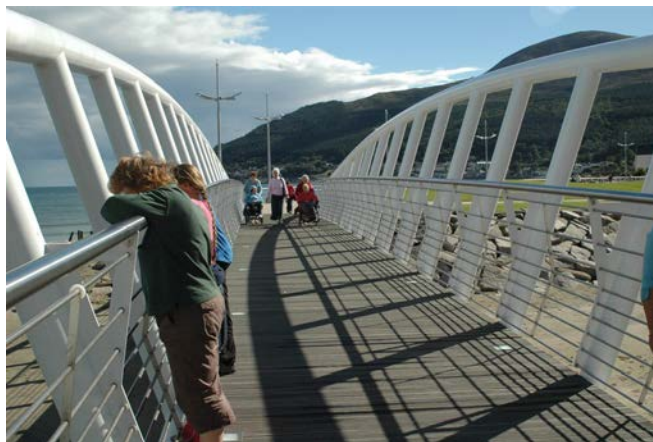
Figure M - Vierendeel Arch Bridge Deck
