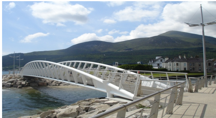
Figure L - Vierendeel Arch Designed by URS
