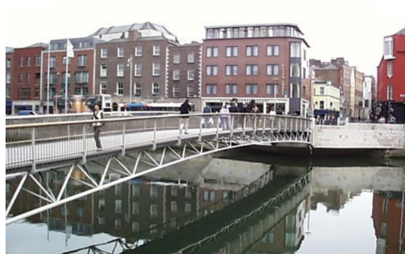
Figure F - Tapered Truss (Millennium Bridge)
