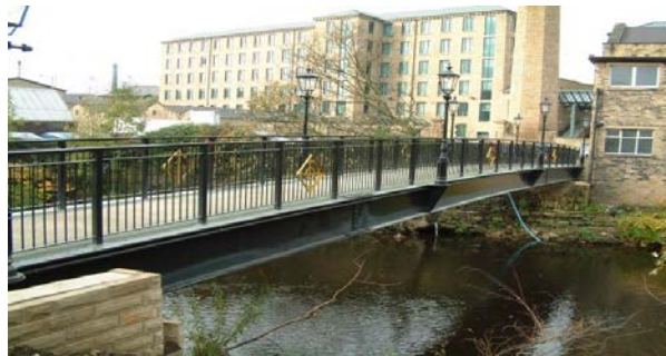
Figure B - Typical Beam Bridge (Birmingham)
