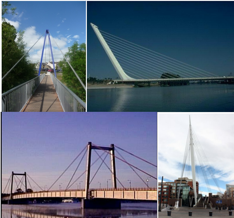
Figure S - Pylon Arrangements
