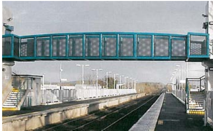
Figure O - Typical Vierendeel Truss (Monasteriven)
