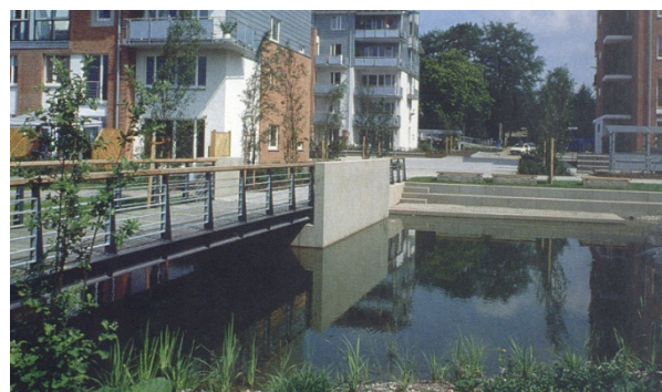
Figure C - Short Span Beam Bridge (Germany)
